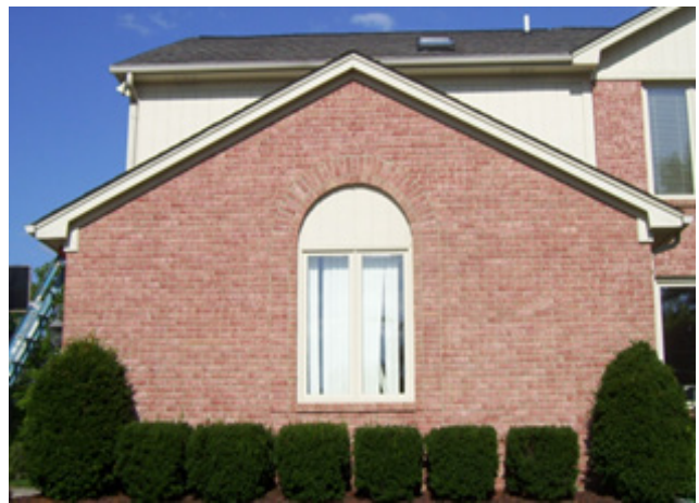
Photo 2 After Staining Applied
