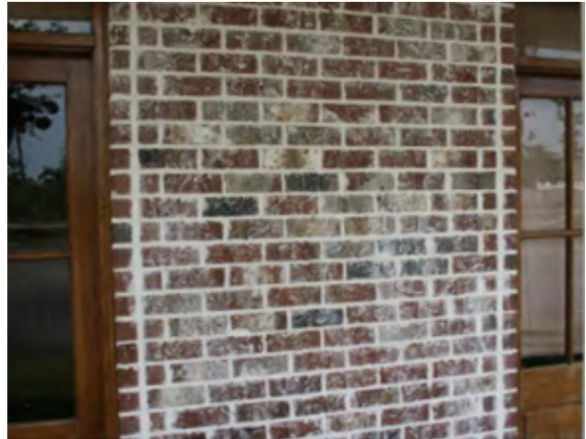
Photo 7 Semi-Opaque Application of Mortar Wash
