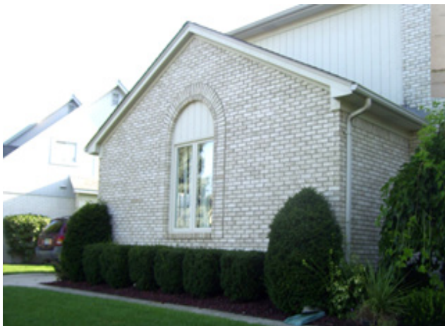
Photo 1 Before Staining Applied
