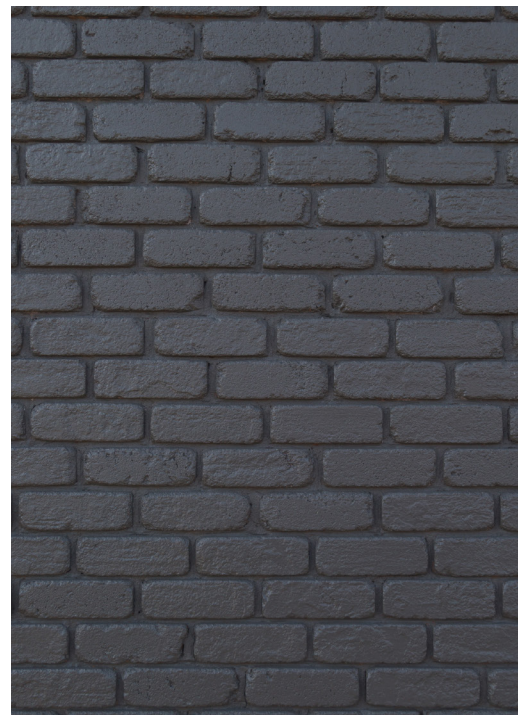
Photo 5 Mineral Paint Finish on Brickwork with Raked Joints
